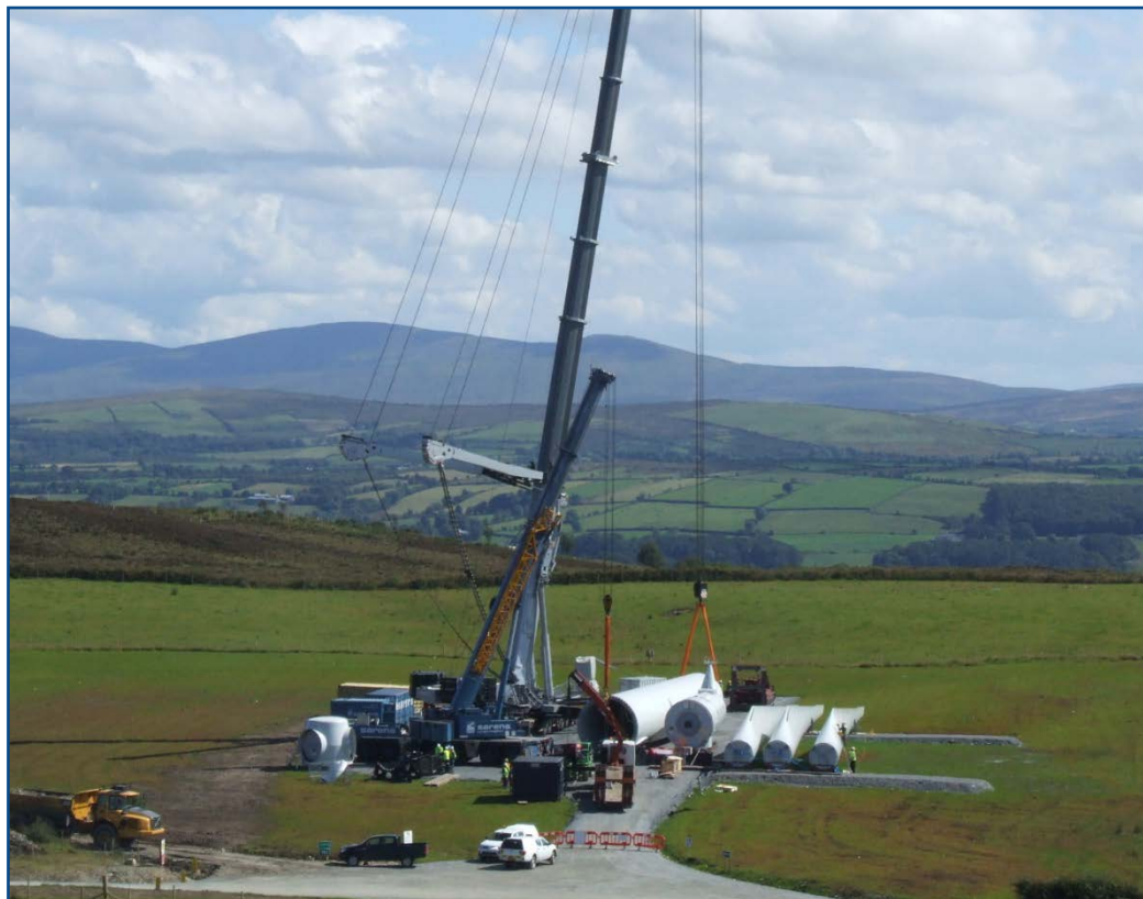
Figure 3.4: Wind Turbine Erection
