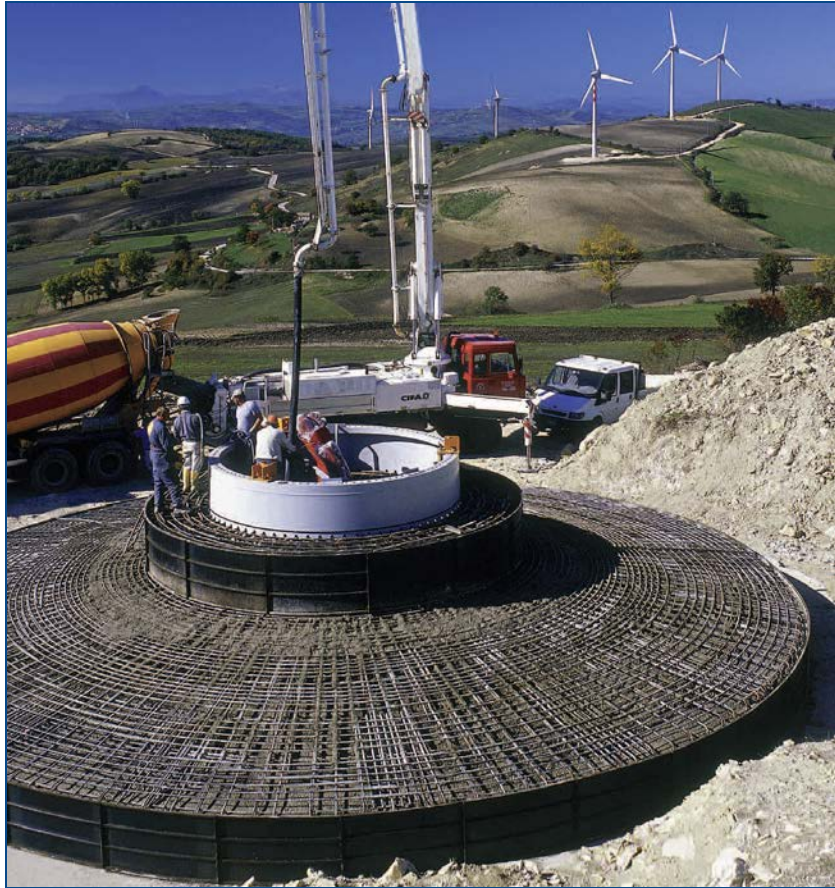
Figure 3.1: Wind Turbine Foundation
