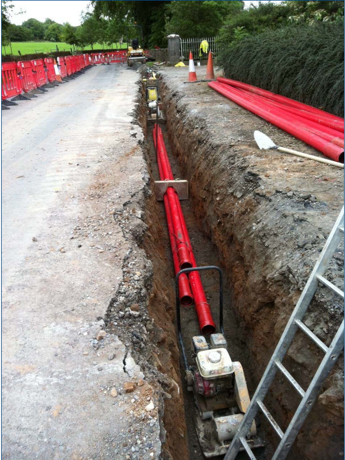
Figure 3.5: Typical 110 kV Cable Installation
