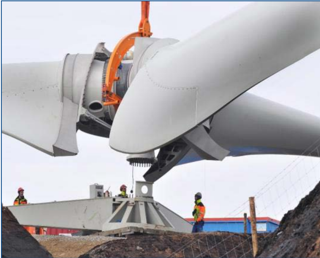
Figure 3.3: Assembly of Wind Turbine Blades
